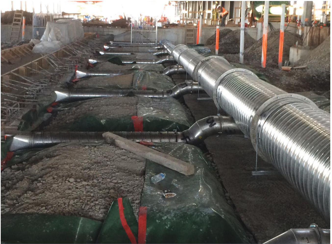
INDUSTRIAL: Tam-Kal follows the strict Sheet Metal and Air Conditioning Contractors' National Association (SMACNA) Industrial standards and uses G90 dry passivated metal. PHOTO COURTESY OF TAM-KAL
